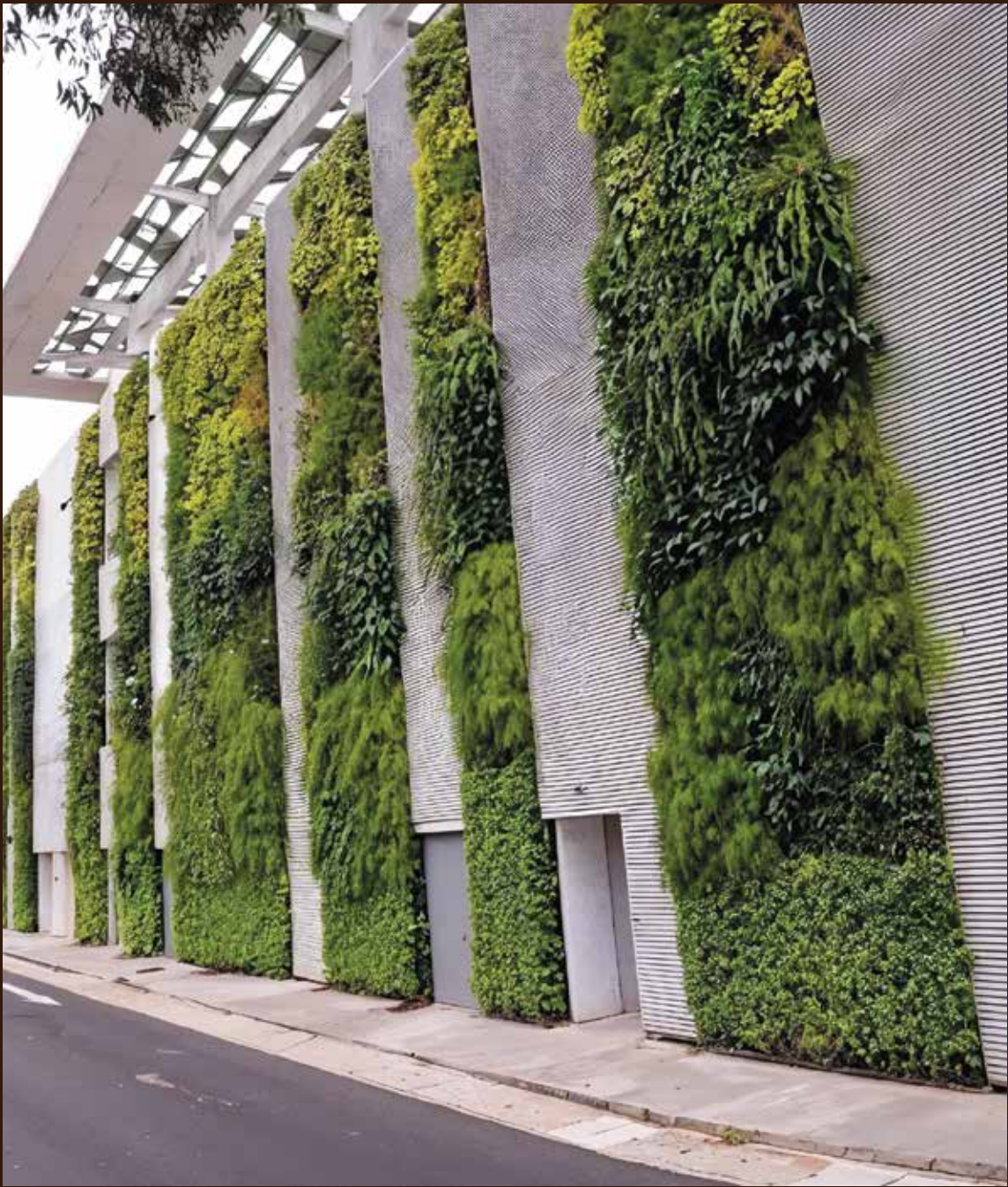
Vertical Green Wall
